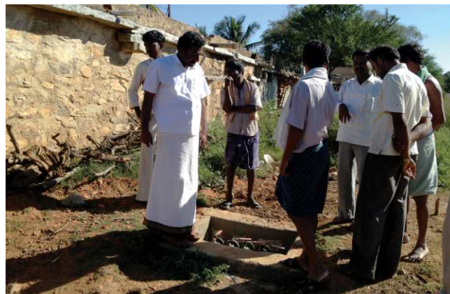
GP members inspecting the system for equal drinking water distribution
